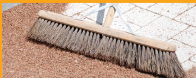
Surface Dressing 2-4mm clean crushed stone
